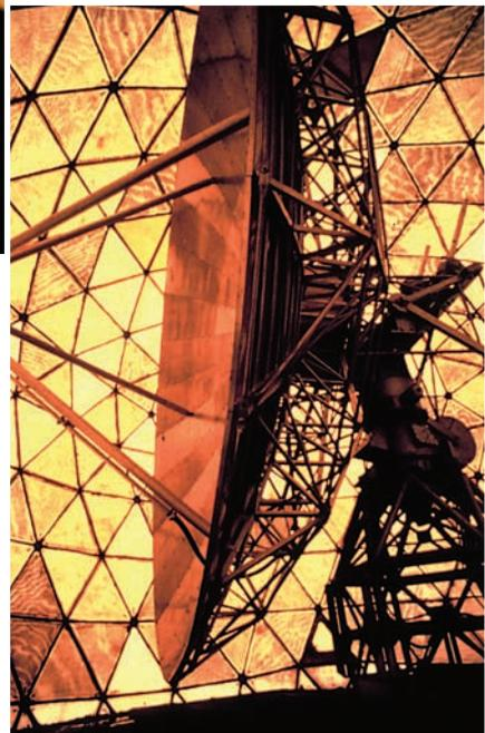
*Meteorologists have many tools for gathering information. Among the most effective is Doppler radar, capable of showing squall lines and other weather features moving through an area.*
